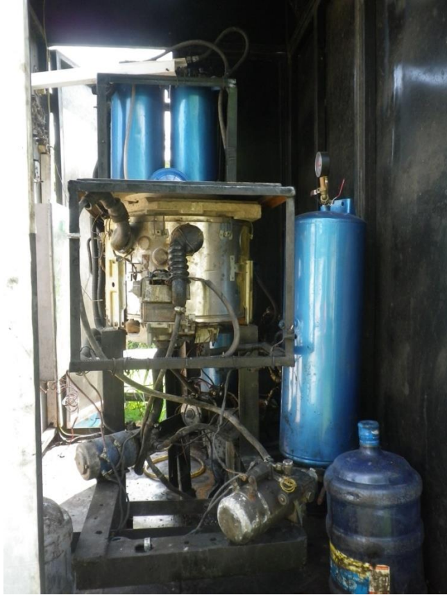
Plate 4: Flash Still to the right-hand side of Centrifugal Contactor Separator
